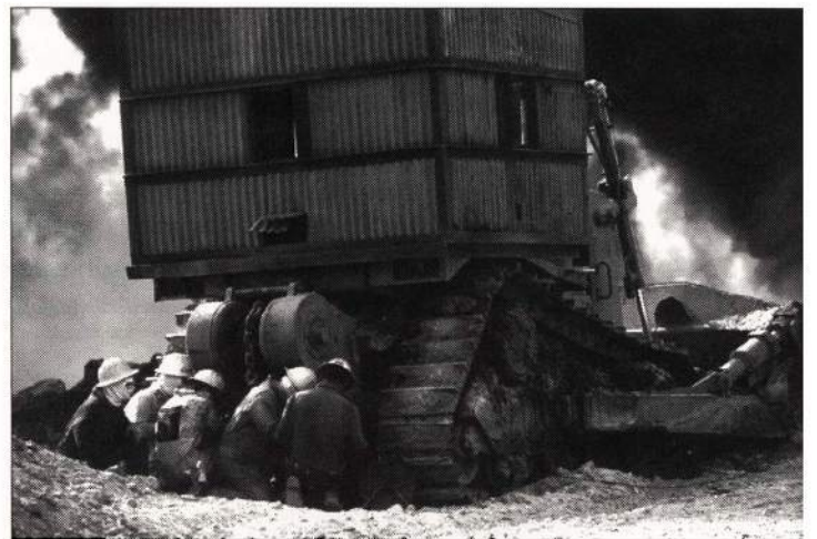
A Texan firefighting team takes cover when dynamite is used to dislodge built-up coke from the well head.
