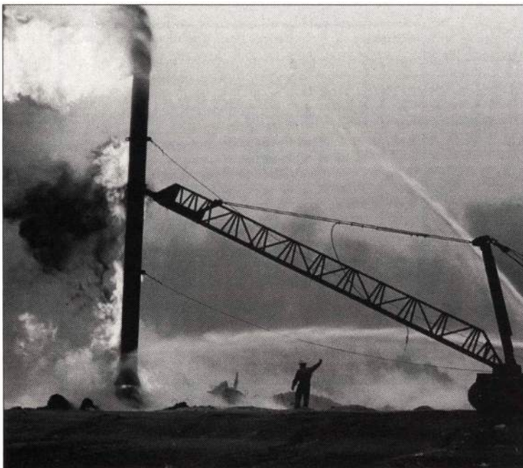
The Wild Well Control team backs a stinger towards well. Monitor sheds in the background shield the firefighters from the intense heat.
