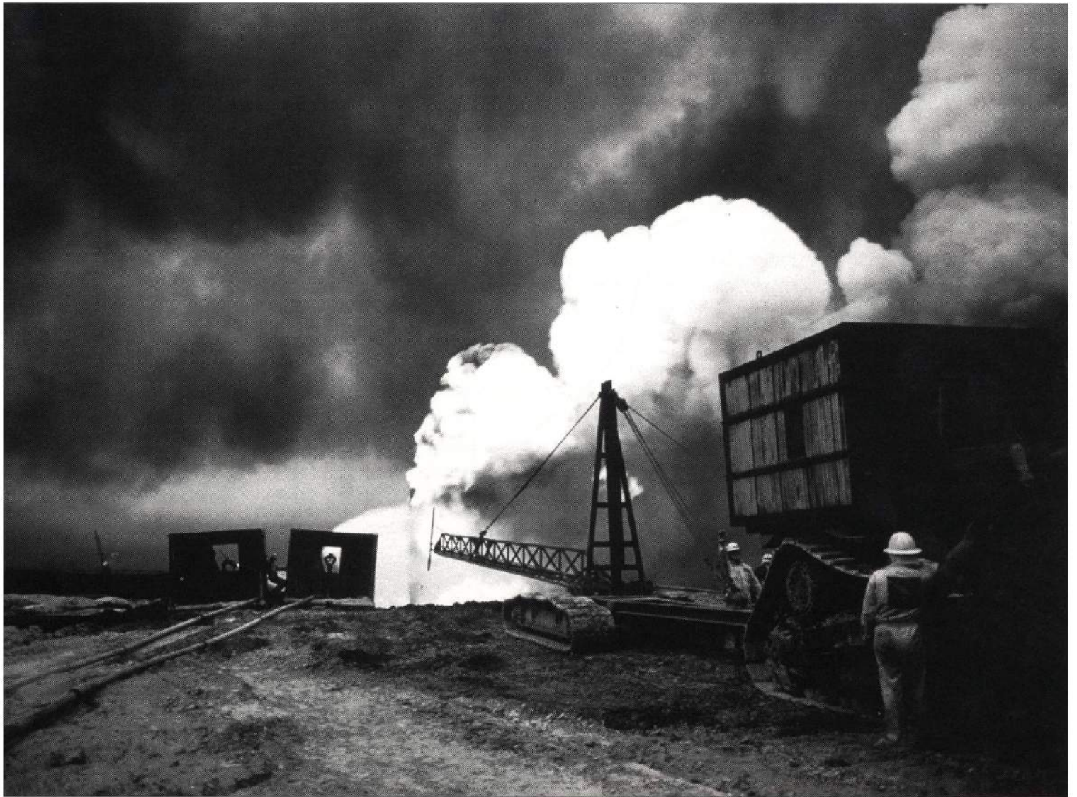
The Wild Well Control team backs a stinger towards well. Monitor sheds in the background shield the firefighters from the intense heat.
