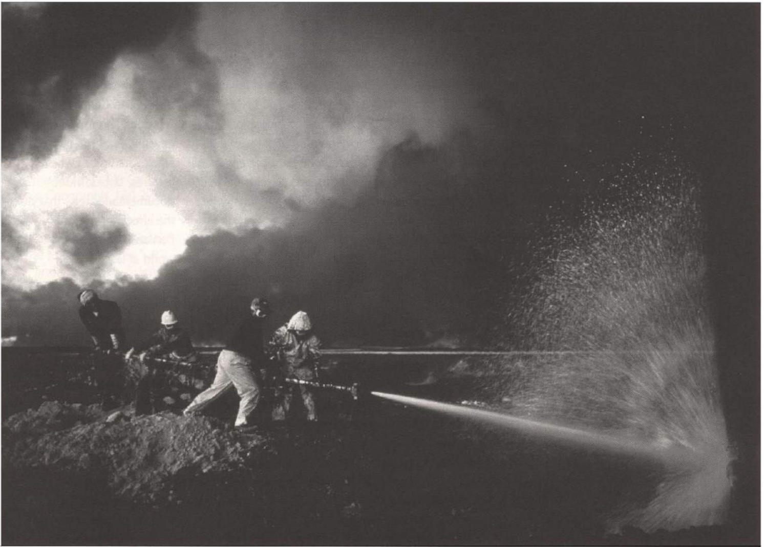
The Kuwaiti team wrestles with a high pressure water monitor to blast baked on "coke" away from the well head.
